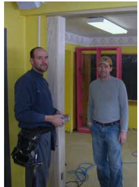
Parishioner & Nursery Remodeling Contractor John Brunner & Associate
